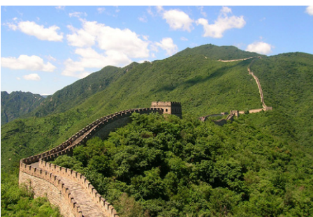
The Great Wall of China
